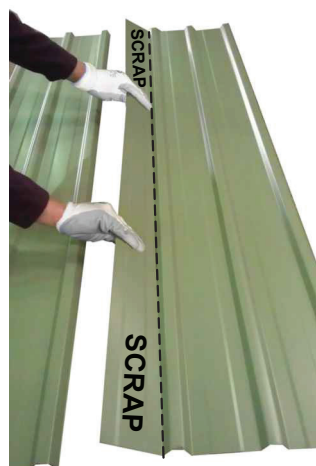
Fold middle section of sheet until free
